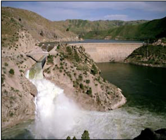
File photo of Arrowrock Dam
