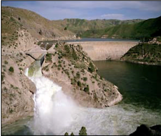
File photo of Arrowrock Dam
